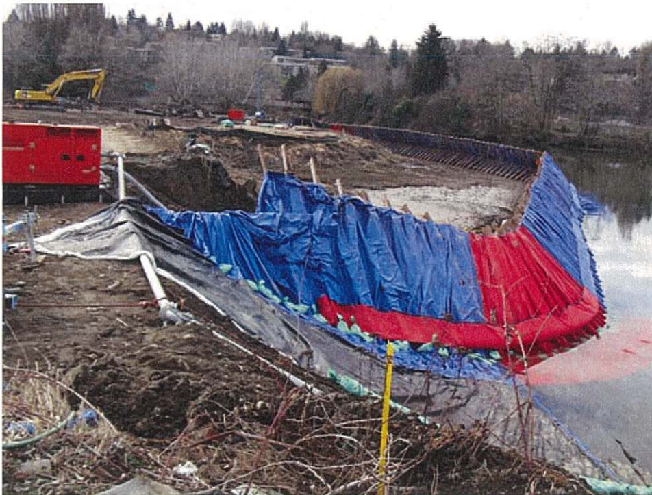
Figure 9 - Photograph of a Cofferdam Drainage Crossing Method.
