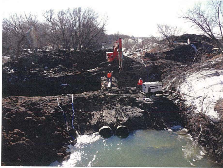
Figure 3 - Installation of Pipe Using the Single Dike Method, Vermillion River.
