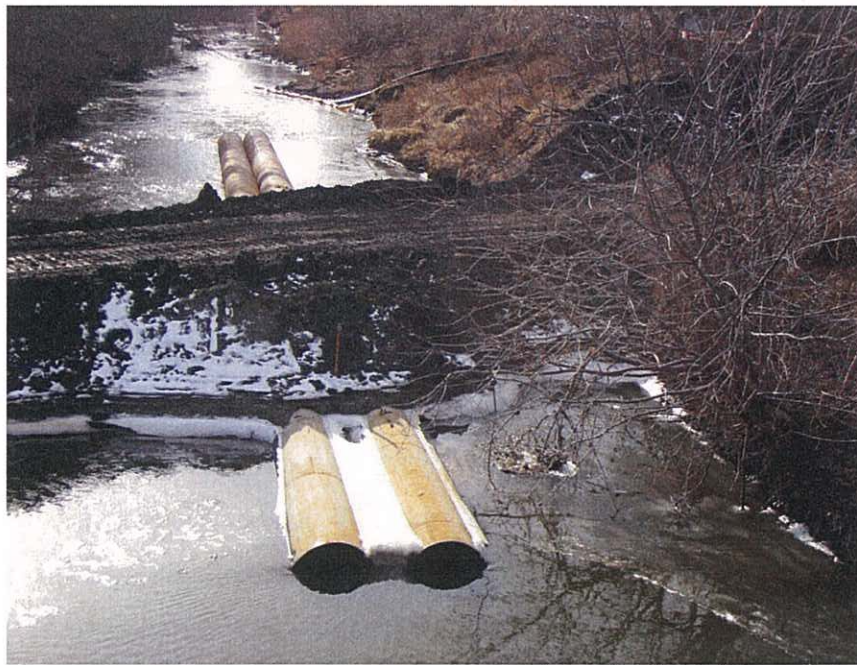
Figure 2 - Single Dike with Diversion Crossing Method, Vermillion River Crossing.
