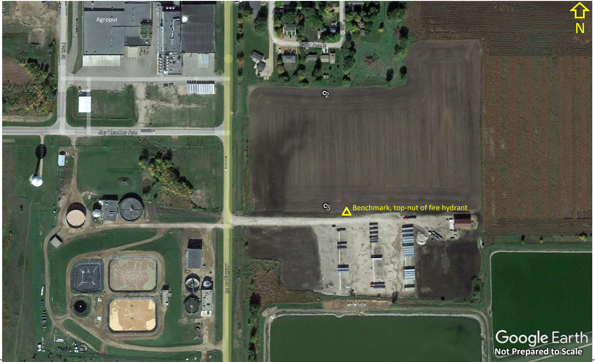
Test Boring Location Image 2 Wastewater Improvements Lake Norden, SD
